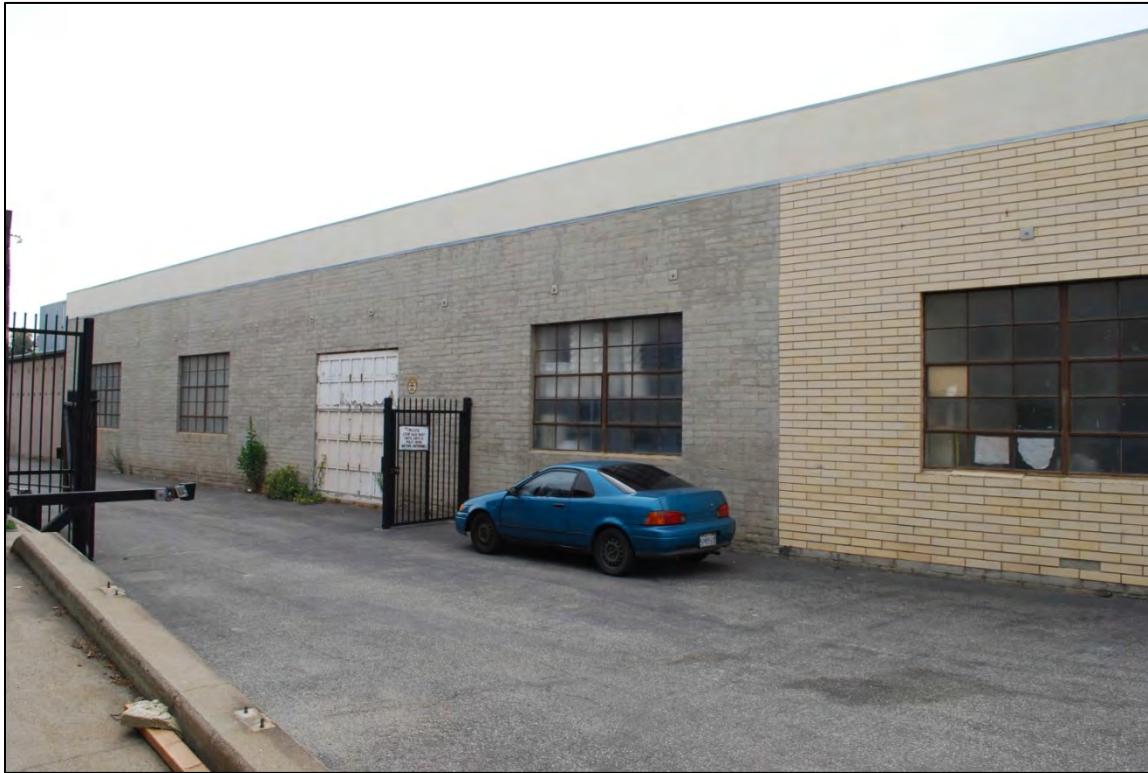
Photograph 5. Overview of north elevation (view to the south)
