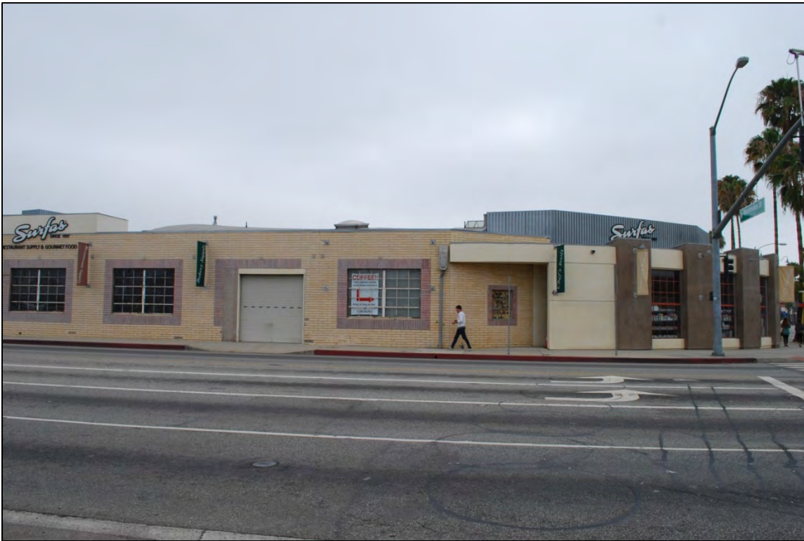
Photograph 1. Overview of west elevation (view to east)
