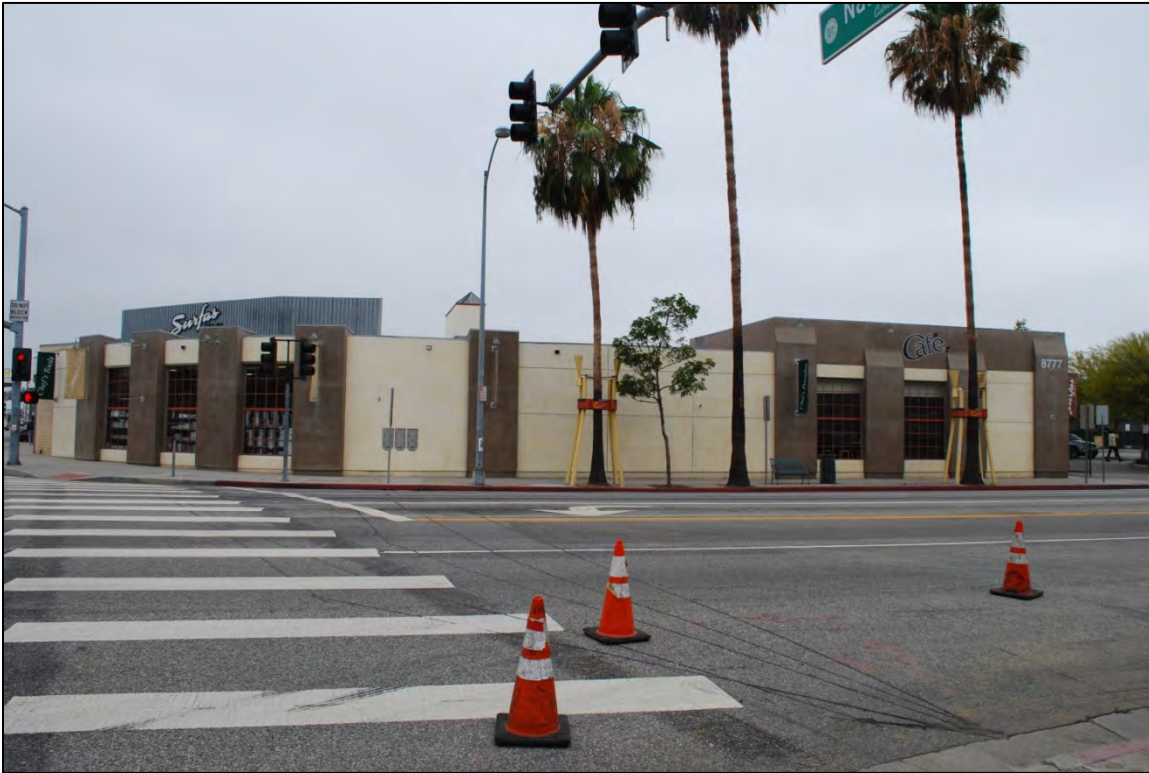
Photograph 3. Overview of the south elevation (view to the north)
