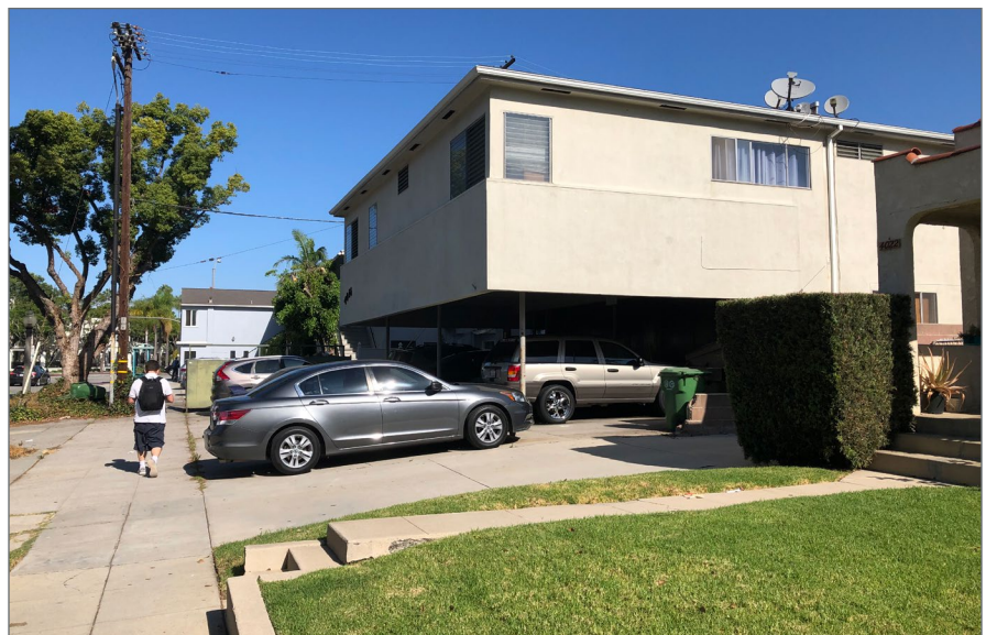
Apartment building with soft-story in Park East neighborhood
