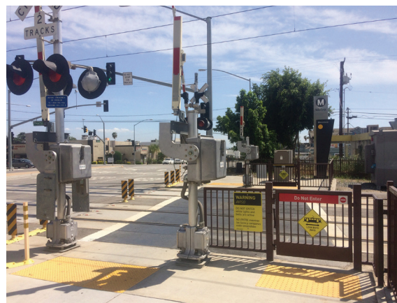
Safety elements of a gate and pedestrian arms have been constructed at the Monrovia Station.
