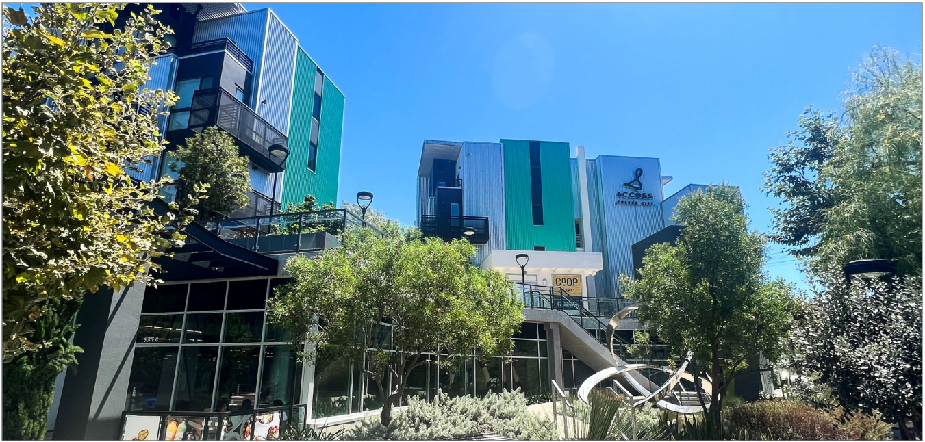
Access Culver City mixed use residential development—LEED Silver
