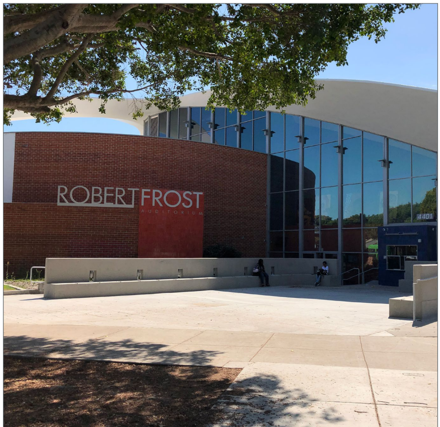
Robert Frost Auditorium at Culver City High School
