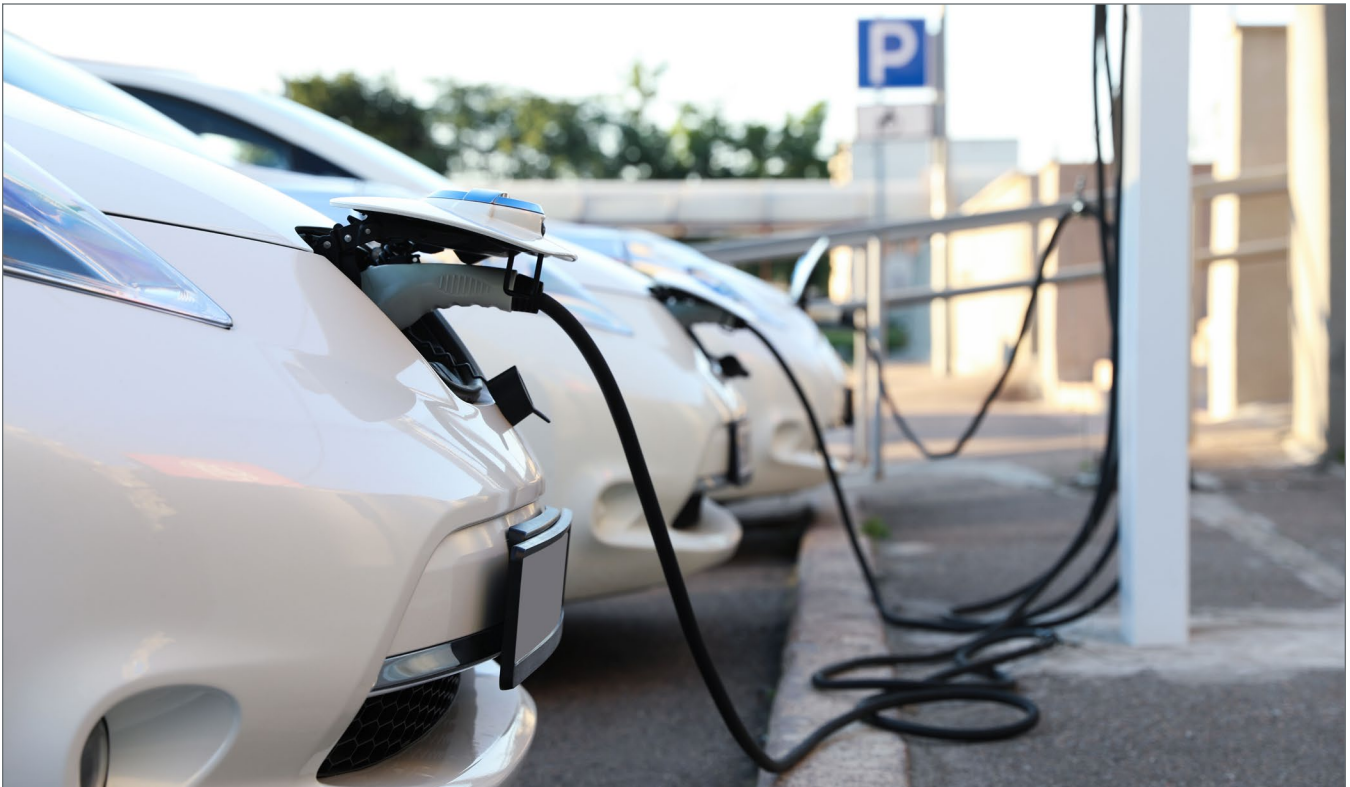
Electric vehicle charging
