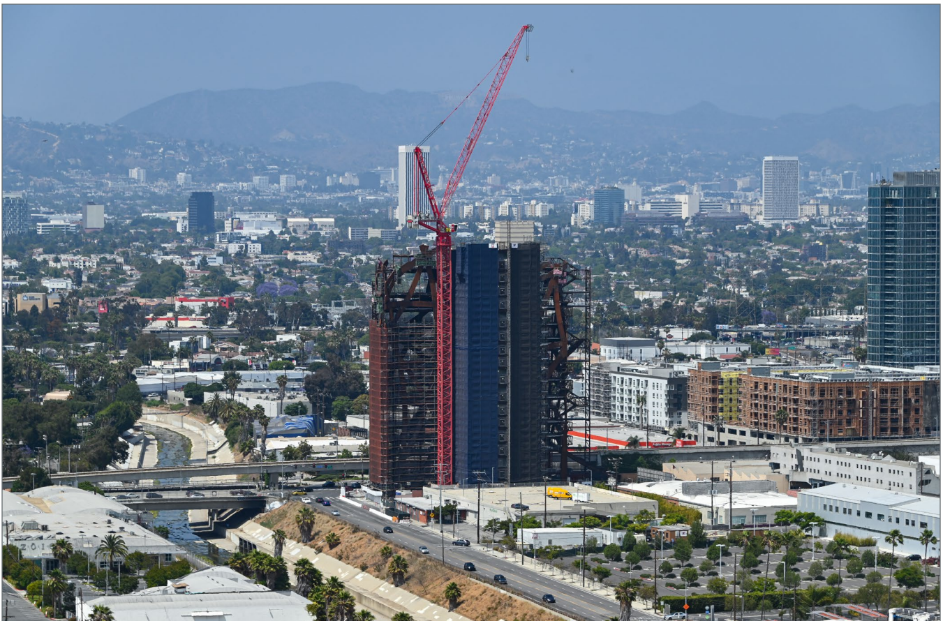
New construction near Culver City
