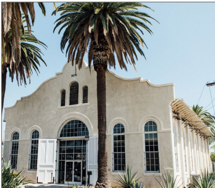
Exterior of Ivy Substation
